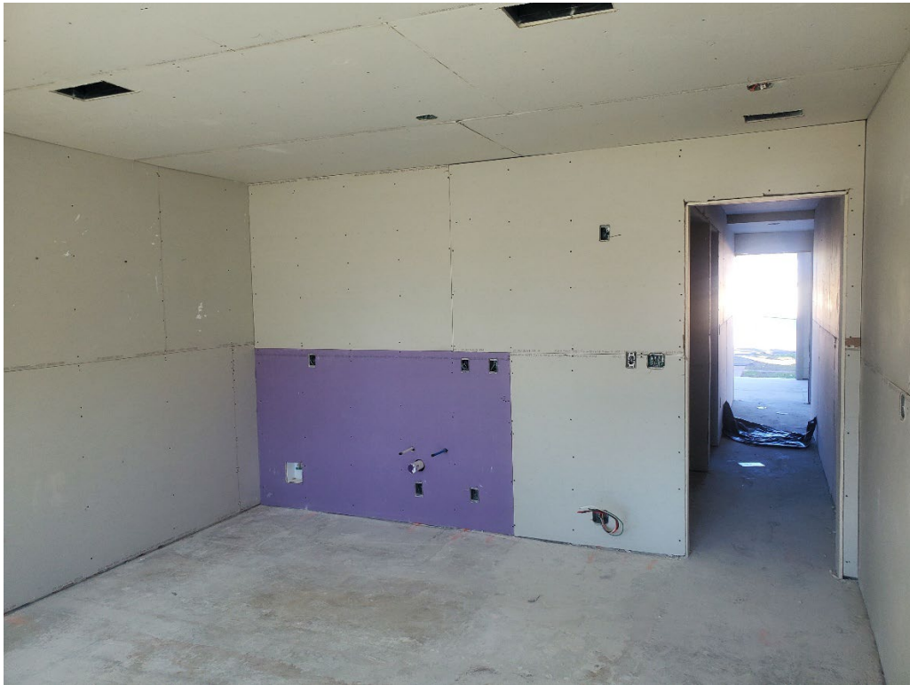
Typical unit interior, east tower
