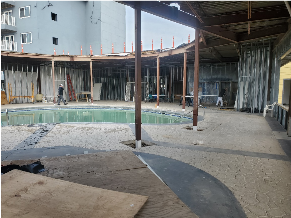
MAIN COLUMNS HAVE BEEN REPAIRED AND EPOXY COATED FOR BELOW GRADE PROTECTION
