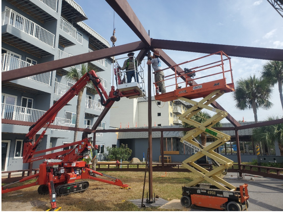
CONSTRUCTION PROGRESS OF PENTAGON STRUCTURE
