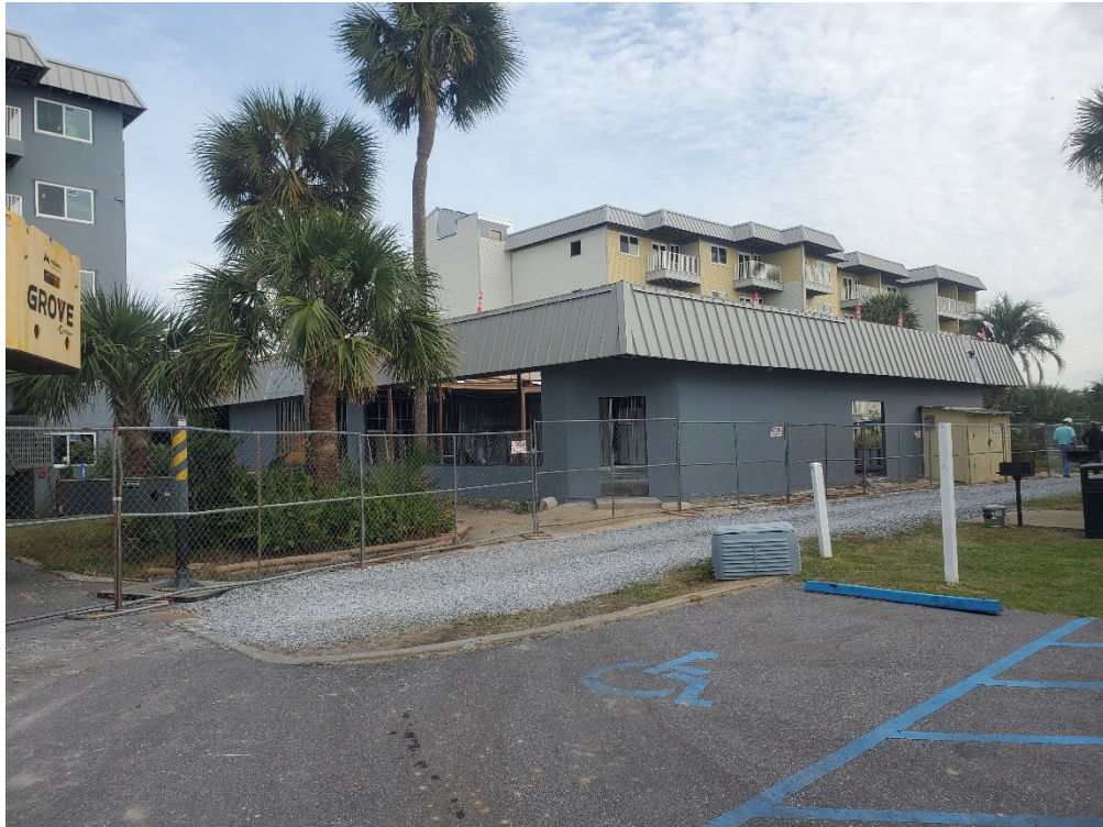
REC BUILDING READY FOR WINDOWS, DOORS, AND PENTAGON
