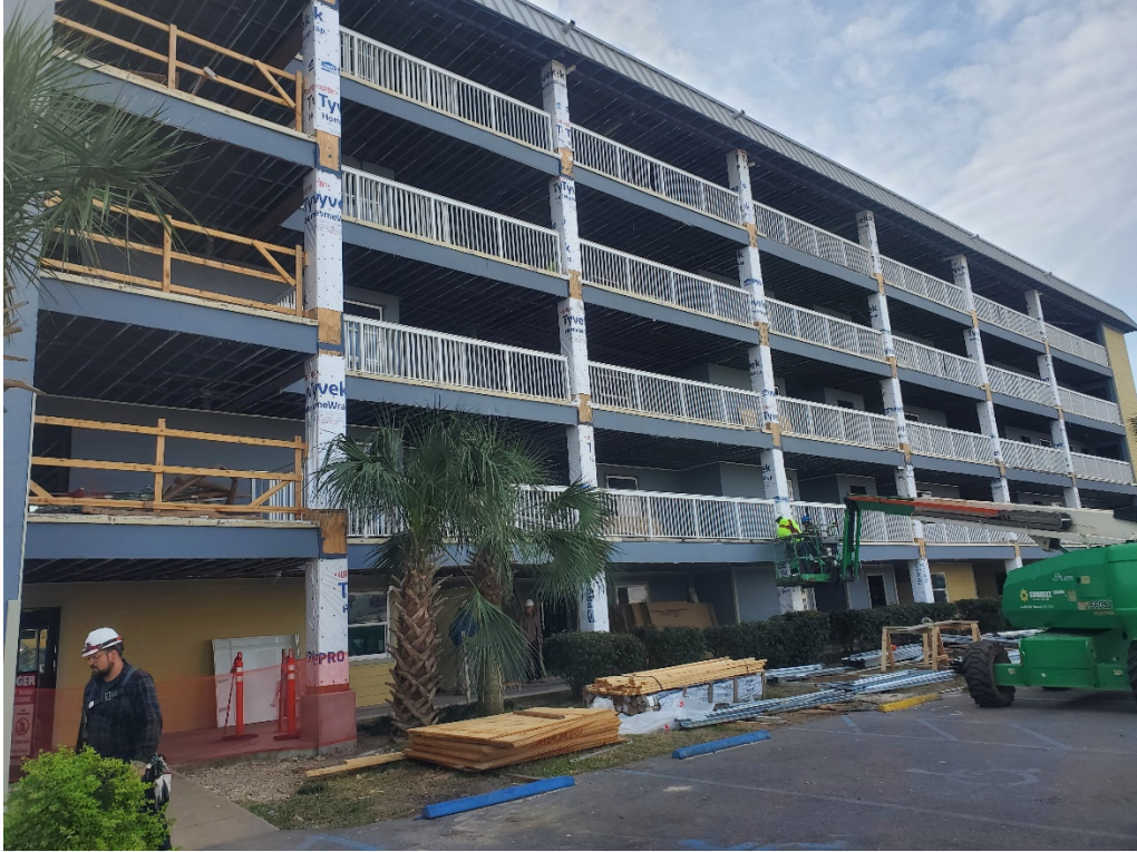
NORTH ELEVATION OF WEST TOWER
