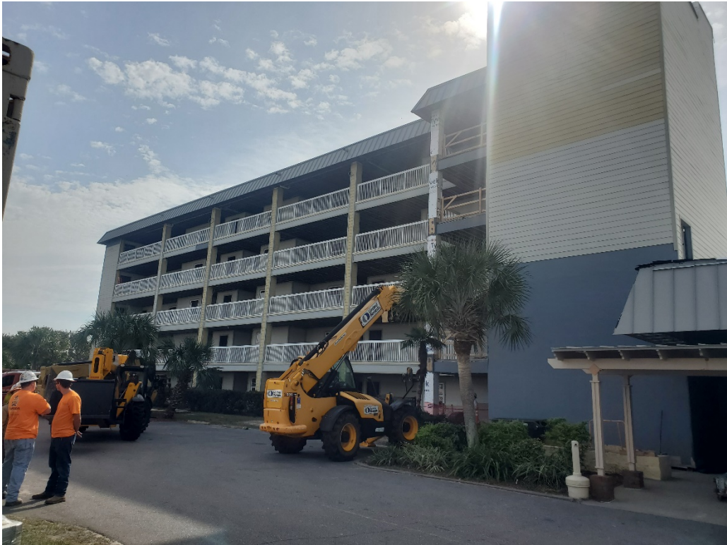
NORTH ELEVATION OF EAST TOWER
