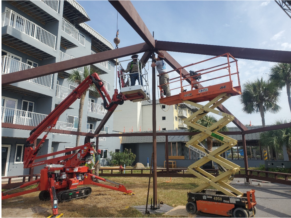
CONSTRUCTION PROGRESS OF PENTAGON STRUCTURE
