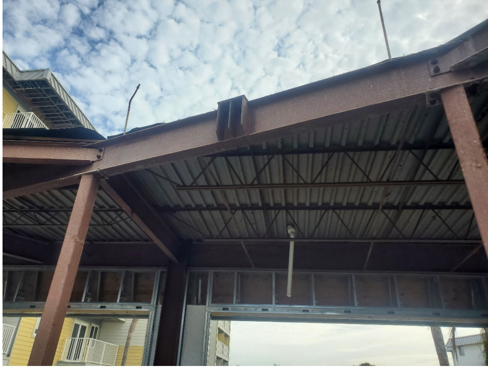
MODIFICATIONS MADE FOR NEW STRUCTURE ATTACHMENT
